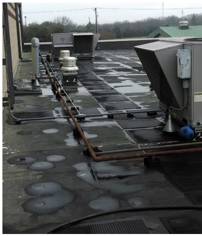
Before GacoFlex S20 was applied.
