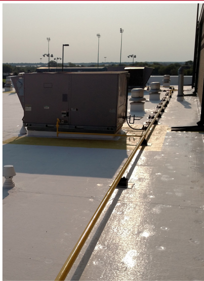
After GacoFlex S20 was applied.
